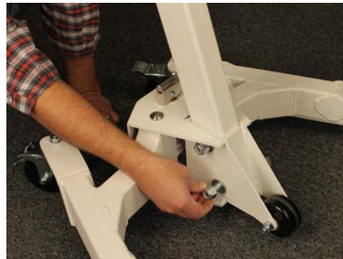
Install Bolts, Washers & Nuts
